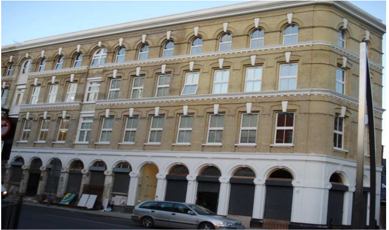
44/48 Commercial Street, LONDON, E1 6LT. We have done the interior design of this project. We were also the structural engineer for renovation of this beautiful building. Client: Dr. Nanda, Nanda Group Ltd
