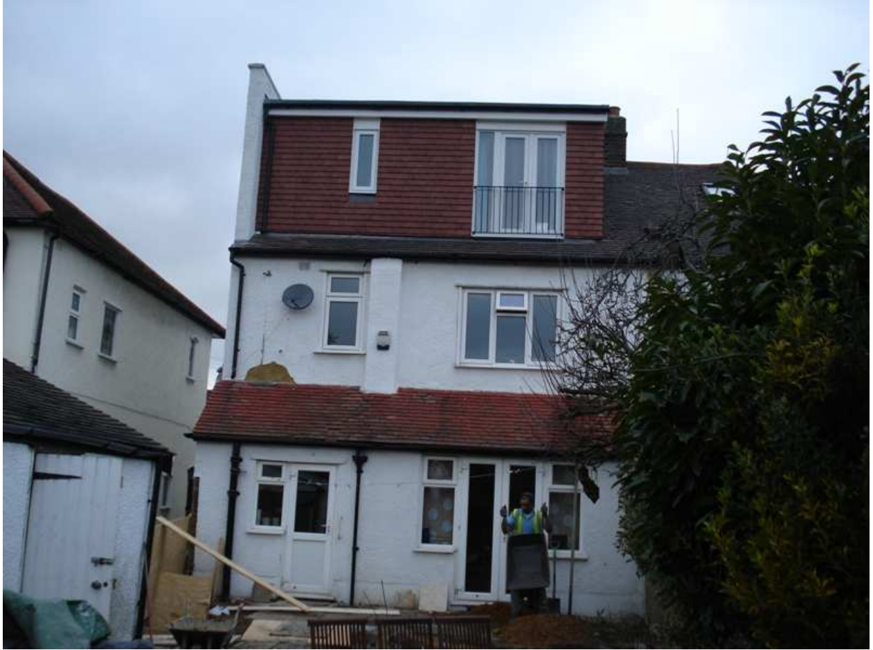
132 Longwood Gardens, Ilford, Essex, IG5 0BD. We were the designer and structural engineer for full dormer loft conversion for this semi-detached house. Architectural services for rear extension have been done by us too. The rear extension is not shown in this photo. Client:- Mr. Rahzeb Chowdhury
